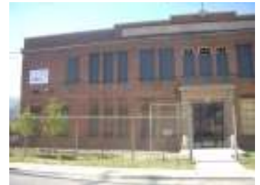
New plywood in the window openings protect from the cold
