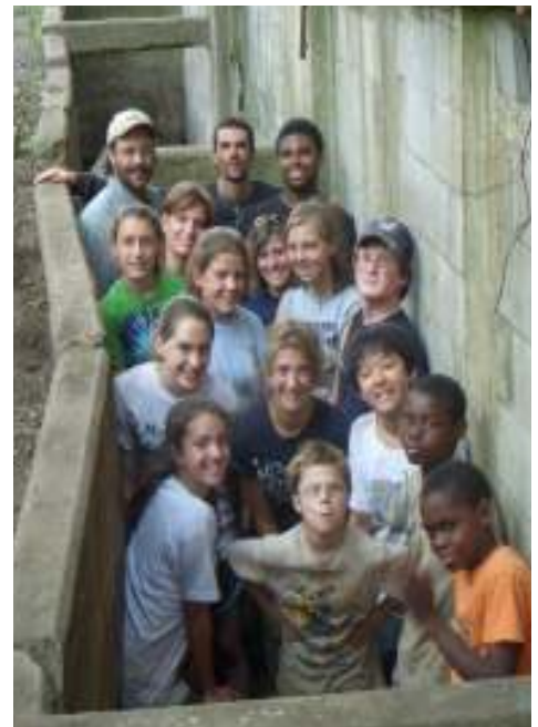
The first window well to be emptied!
